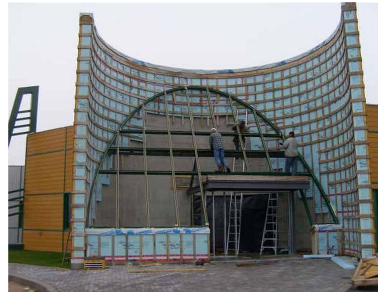
New Wemindji CMC under construction, June 2015
